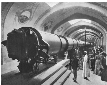
Fig. 25 The Great Paris Exhibition Telescope of 1900, with an objective lens of 1.25 m (49 in) in diameter, was the largest refracting telescope ever constructed. It was built as the centerpiece of the Paris Universal Exhibition of 1900. 200 ft long. Too big to use.
